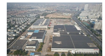
Bird’s-eye view of the SOCC plant
