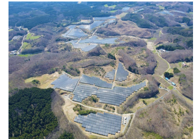
Samegawa Aono Solar Power Plant
